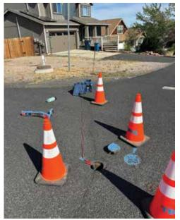
Figure 1 Direct Connection method used to directly apply signal current to tracer wire. (only 2 mA achieved)
