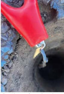
Figure 3 Locator confirms metal to metal connection is made between connection clip and copper tracer wire.
